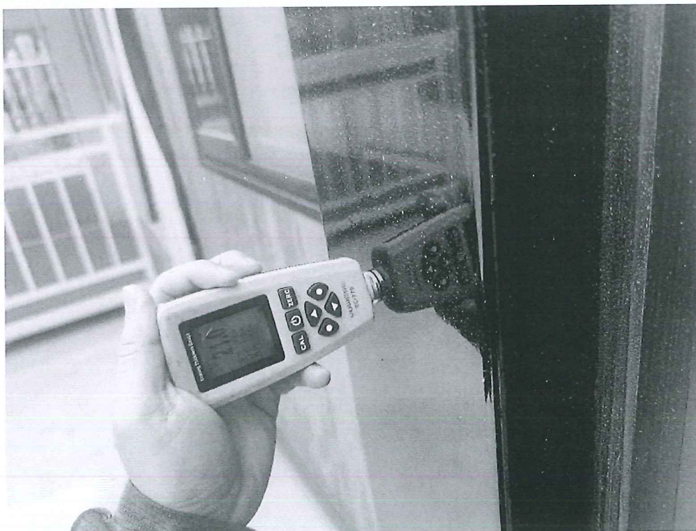
Coating Inspection of Steel Components in Steel Plate House
