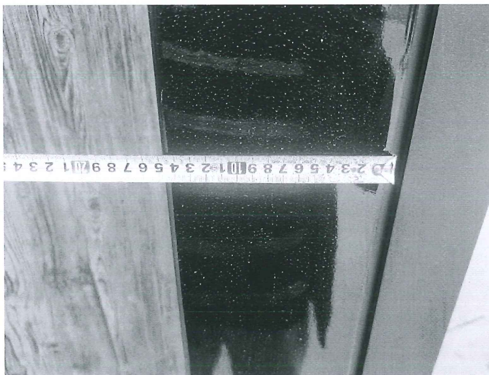
Dimension Inspection of Steel Components in the Steel Plate House
